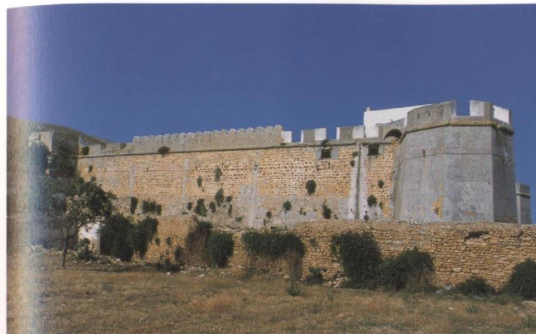
Fort central, tour d'angle, Ghar El-Melh.
